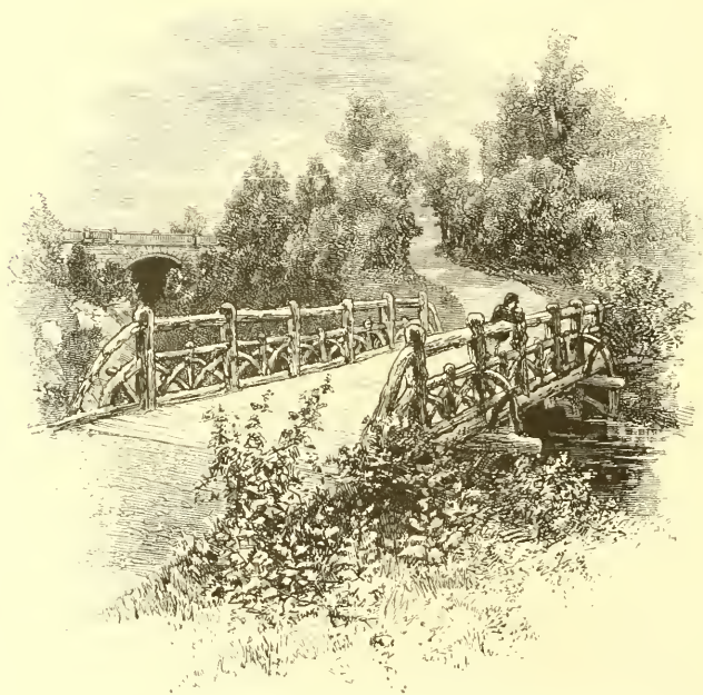
RUSTIC BRIDGE, NEAR BALCONY BRIDGE, LOOKING EAST.
